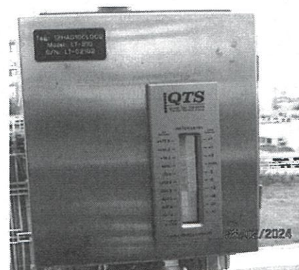
Water Level Indicator on Control Room
